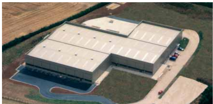
Autogard's modern plant at Cirencester, England
